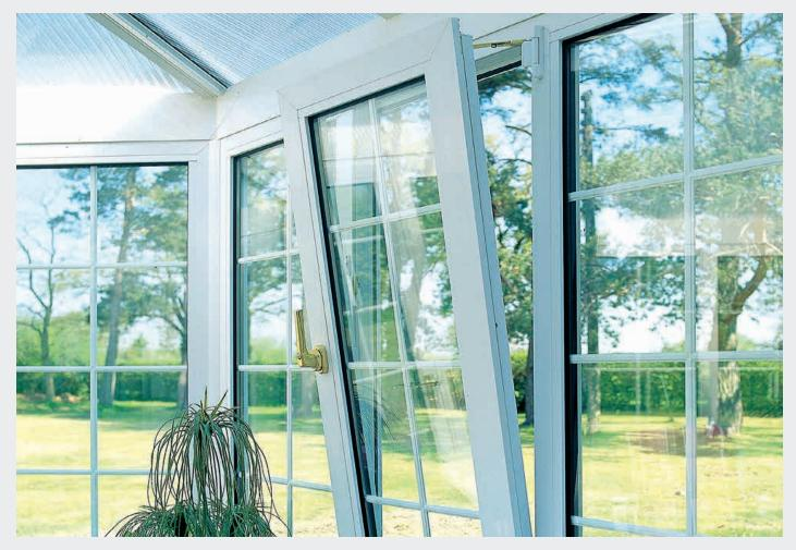
One turn of the handle allows you to tilt the window inwards, then a second turn enables it to open fully inwards for maximum fresh air, an uninterrupted connection to the outside world and ease of cleaning.
